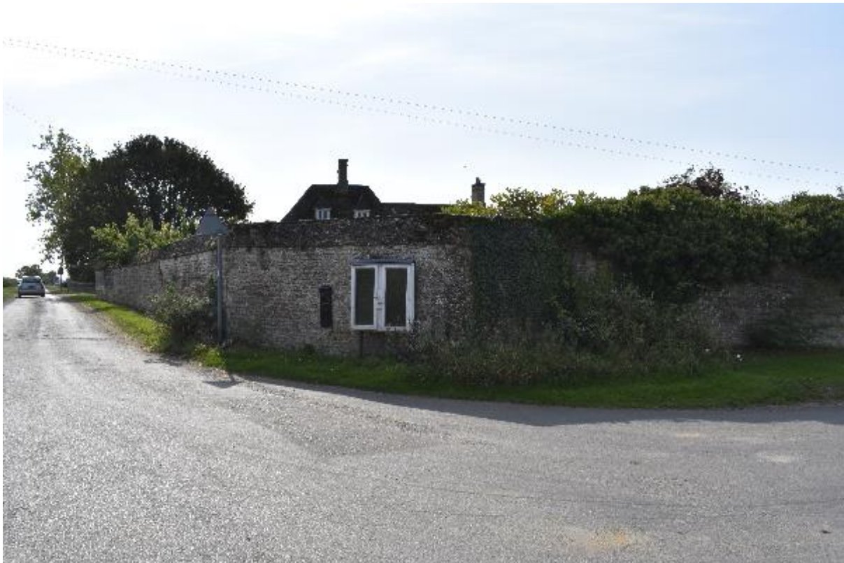
Photo 7 Model Farmhouse and wall, looking south-west
