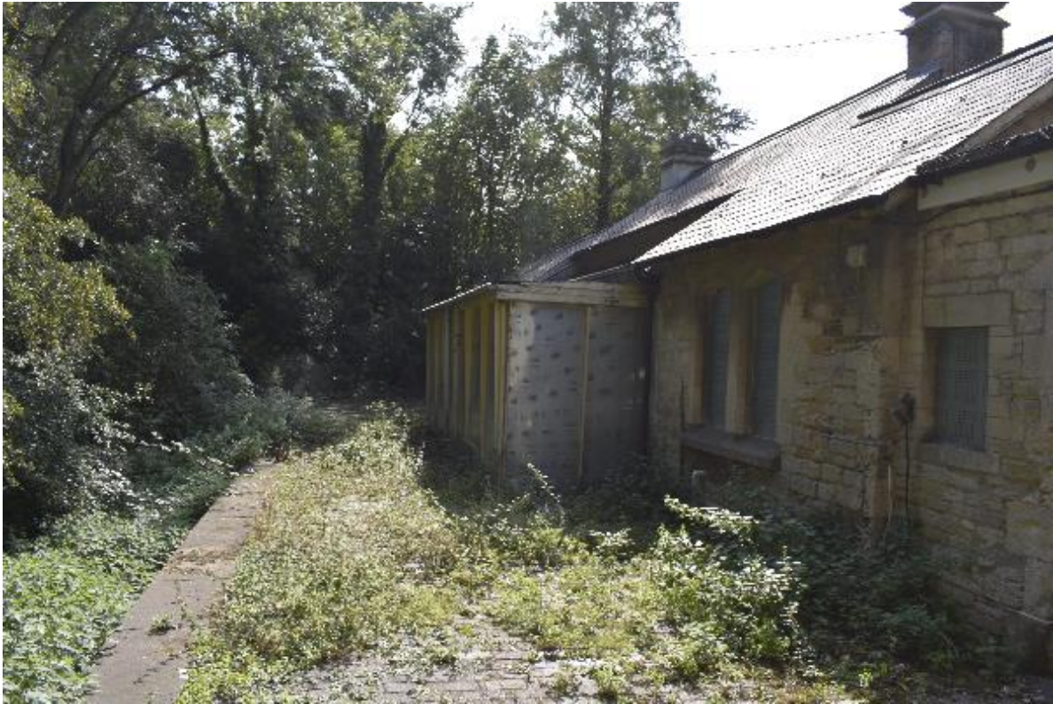
Photo 9 Former station, looking south, showing the platform and platform canopy
