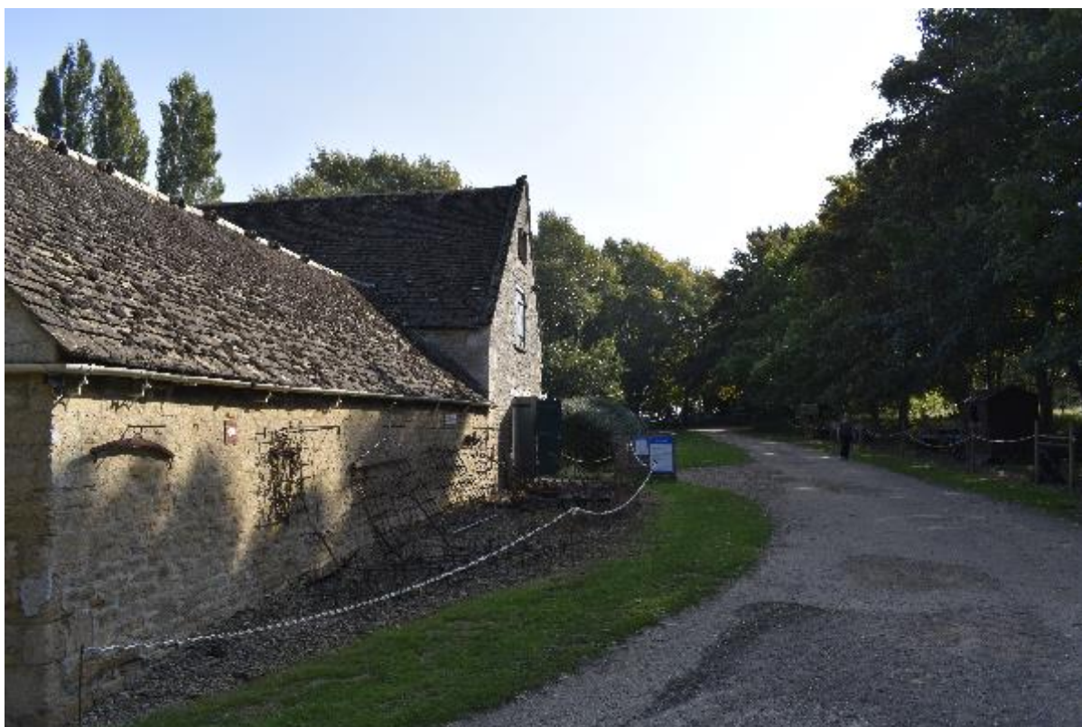
Photo 12 Sacrewell mill, south side of the listed barn, showing the existing access road in the centre-right of frame. The proposed access would tie in to this, minimising change
