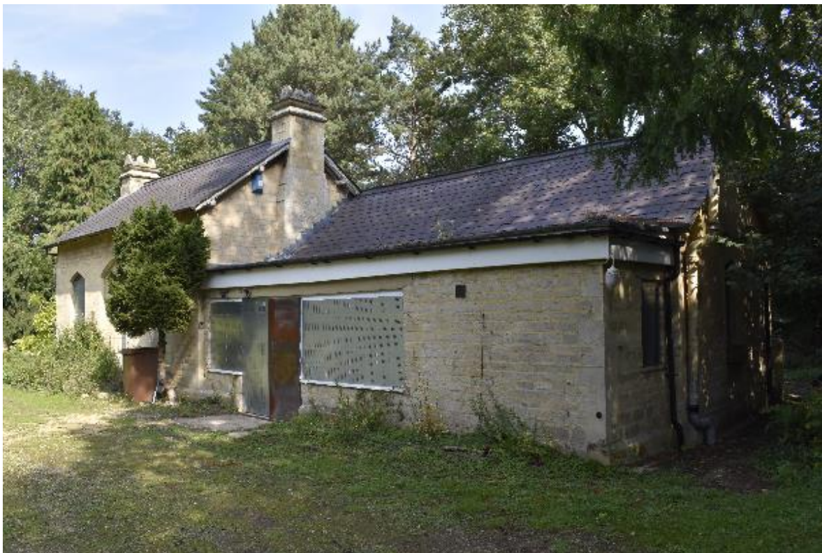
Photo 8 Former station, looking north-east
